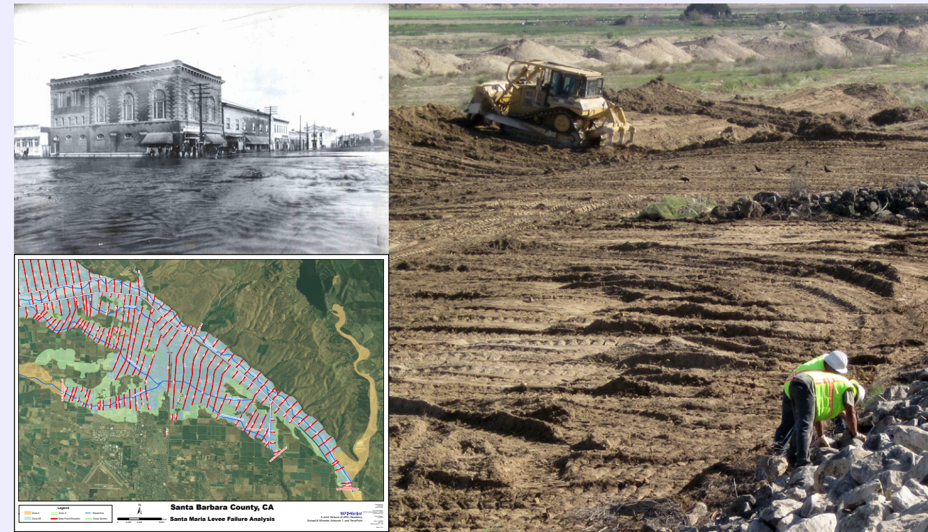
Top left: The intersection of Church and Broadway in Santa Maria during the flood of 1914. Bottom left: The FEMA 2008 Santa Maria Levee Failure Analysis. Right: Clearing and grubbing along the levee—in anticipation of the Army Corps of Engineers levee improvement project, contractors inspect the rock slope protection in January 2010 while a track-type tractor works the river channel.
