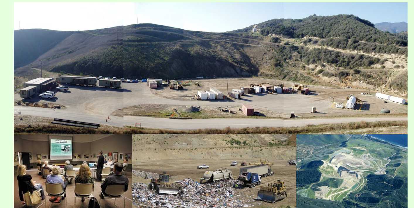
Top: Composite photo of the proposed Conversion Technology site at the Tajiguas Landfill from December 2009. Bottom left: There were over 40 presentations to community groups. Bottom: Local solid trash collectors deliver their waste while a wheel dozer works on leveling it in preparation for it to be covered with soil. Bottom right: An aerial view of the Tajiguas Landfill from March 2009. The County owned and operated landfill is known for its innovative management practices such as being the first landfill in the State to use falcons for seagull abatement. Tajiguas was also awarded the SWANA Silver Award for landfill management excellence in 2001.
