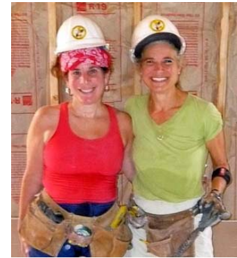
Supervisor Wolf with Karen Heimberg rebuilding church in Alabama
