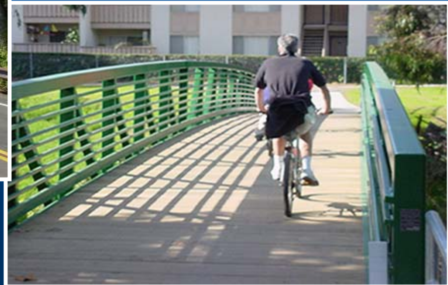
Lassen Bikepath Bridge
