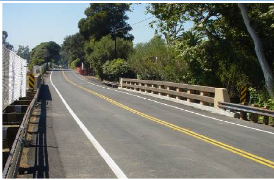
North Jameson Lane Bridge Replacement and Bikelanes
