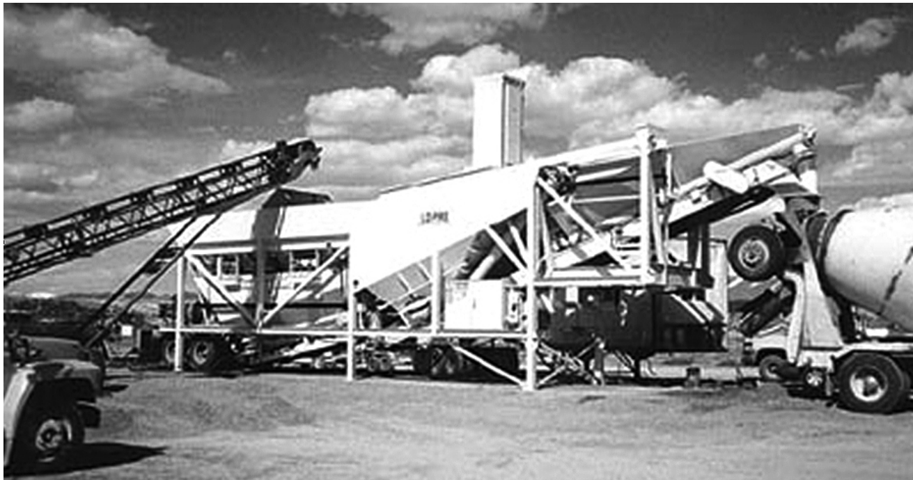
Batch Plant in Operation
