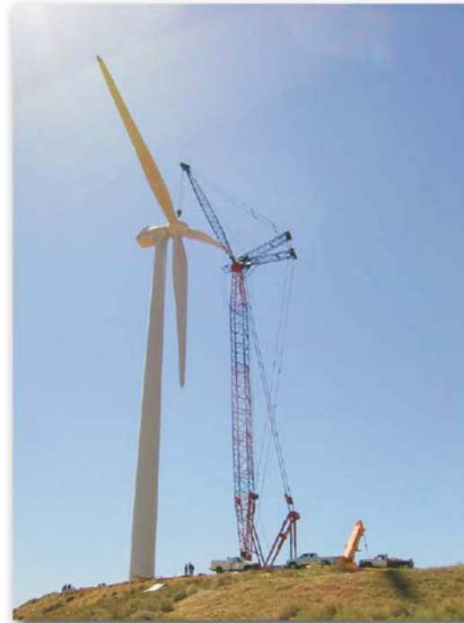
Inset E: Typical WTG construction. The WTG is a 1.5-MW machine. (Photo Credit: Michael D. Burns, Oak Creek Energy Systems Inc., Mojave, California.)
