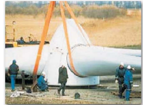
Inset F: WTG blade/hub assembly.
