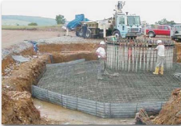
Inset A: WTG Foundation construction.
