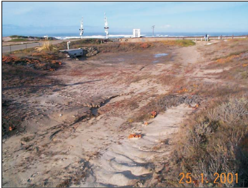
Figures 5.4-2: Example of a Catchment Basin (Basin 1) Adjacent to Onshore Portion of the Pipeline Route. (A weired Concrete Outlet is Shown Near the Upper Left Corner of the Photograph.)
