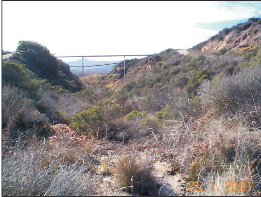
Figures 5.4-1: Photograph of Pipeline Route Crossing Small Drainage Feature Near Basin 4.
