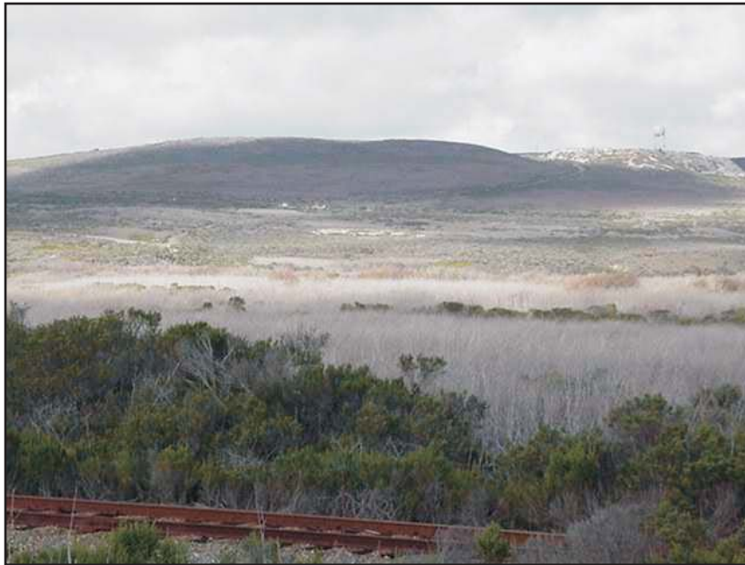
Figures 5.13-6: Route 246 to Valve Site #2 (View Position 5) (View of Surf Substation looking west from the west end of Ocean Avenue. The low vegetation is in the foreground, the substation is in the mid-ground and the ocean is in the background.)
