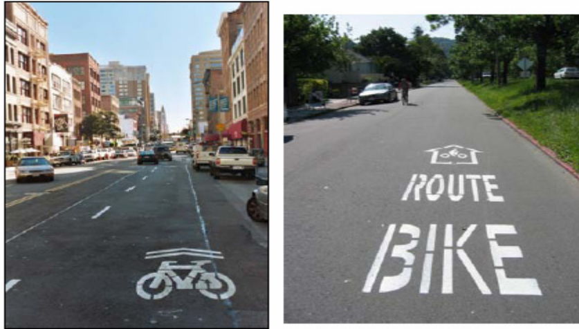
Figure 4.7-2: Examples of Bicycle Boulevard Pavement Markings
