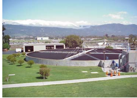
Goleta Sanitary District — Biofiltration Unit
