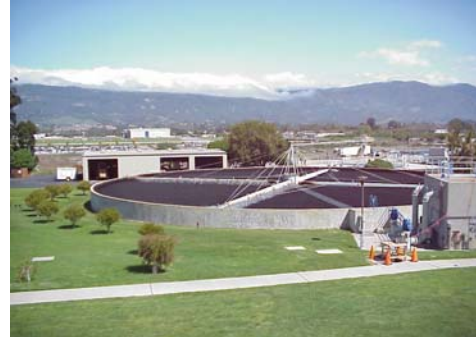
Goleta Sanitary District — Biofiltration Unit
